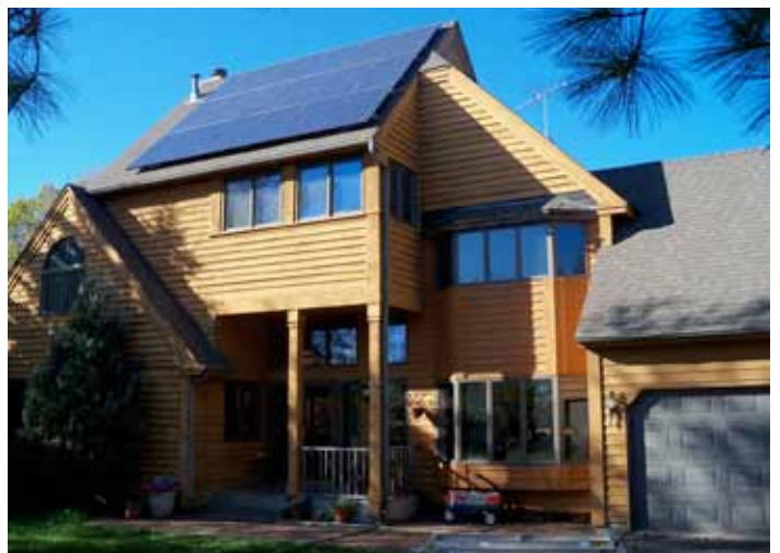
Residential PV solar installation in Minnesota
